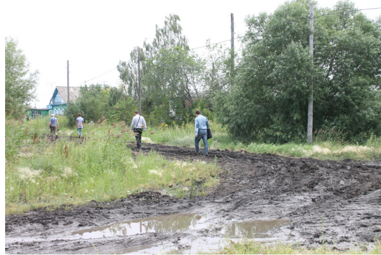
Poor condition of unpaved pads
